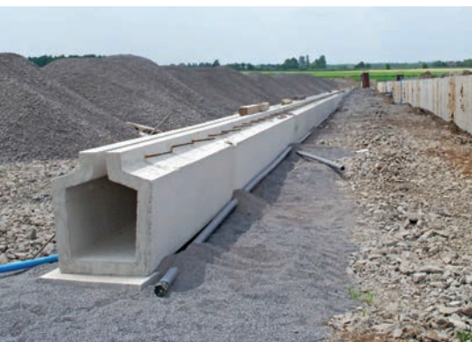
Precast tube sections include gasketed joints and coupling hardware.
