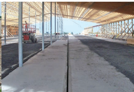
The tubes are backfilled and the alley floors are poured on each side.
