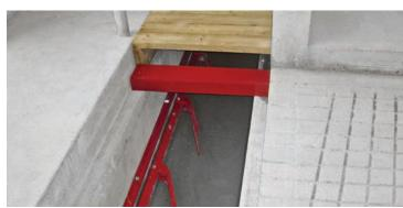
Doing the job right is easy with proper planning. Keyed edges on the cross gutter are ready to accept Jamesway Modular Gutter Covers. The same notch supports light duty walkway covers between the scrape alleys.
